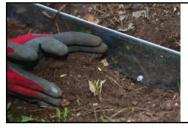
**Tip:** The screw must be under the level of the soil for safety and aesthetic reasons. When using angled stakes, it is necessary to insert two screws at the bottom.
