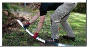
For corners, lay something straight such as a piece of timber, across the edge and lever edging up to create the desired angles. Their are multiple methods of shaping the edging, the best method will depend on the user.
