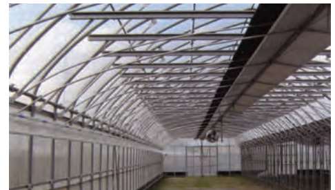
Animal Confinement Structure
