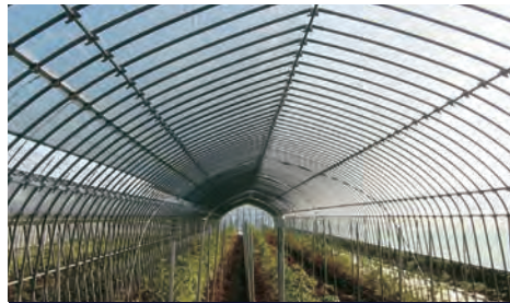
Green House Structure
